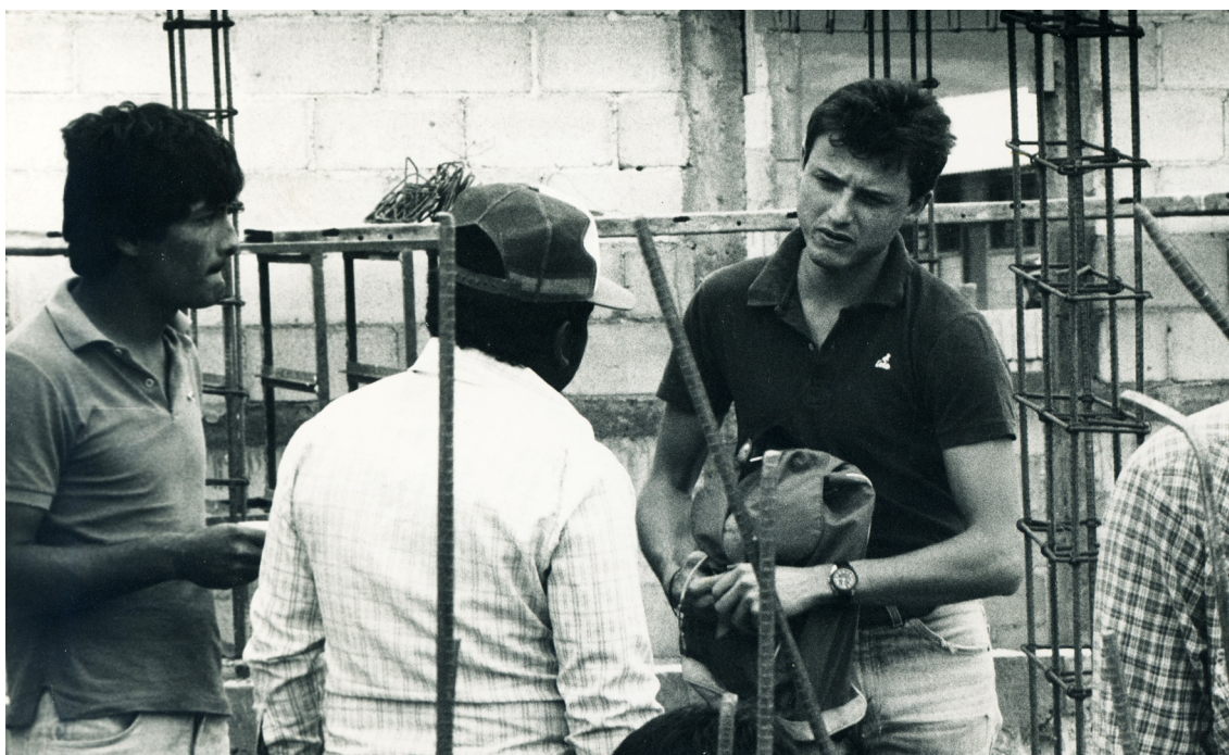
Francisco A. Diaz Lison, in charge of the construction of a medical centre in Guatemala de la Asuncion, 1988
